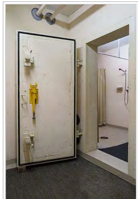
Concrete door of a public fallout shelter in Switzerland (2014).
