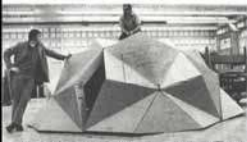
Done to strong enough to support two adults, and light enough for use in heavy. Door gap doesn't seriously weaken structure. Midwest Institute
