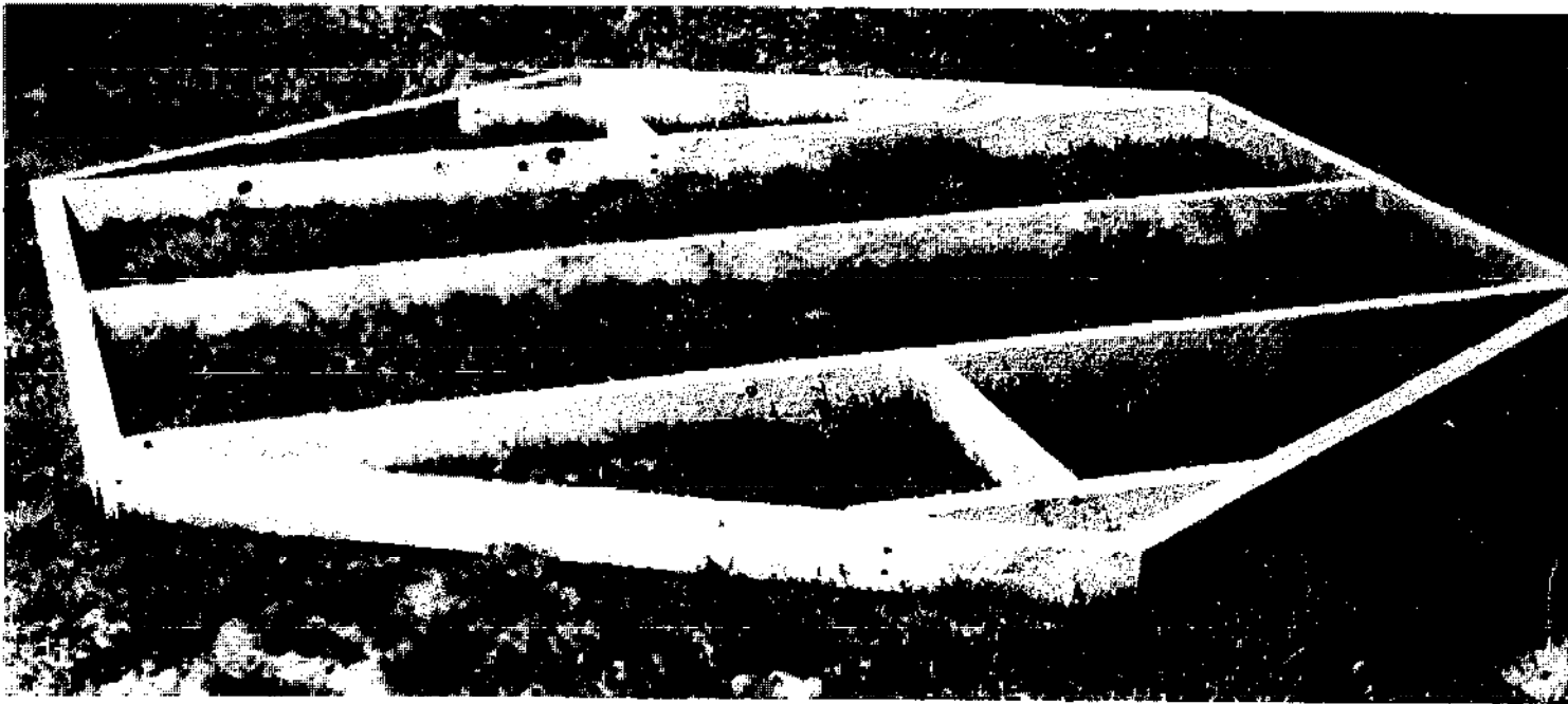
Completed hexagonal foundation for 10-foot yurt.
