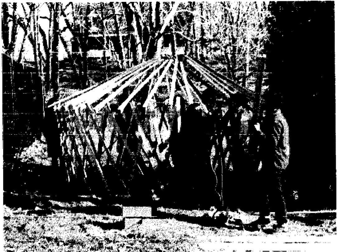
Roof assembly in progress.
