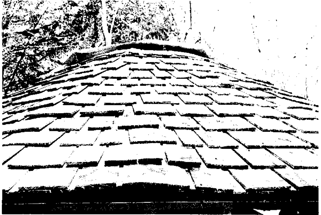
Cedar shingles make an attractive, durable roof covering.
