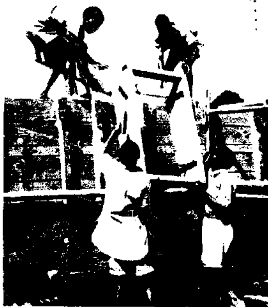
Figure VIII. Forms for Rammed Earth as used in Southern Rhodesia. Note that the window frame is the full thickness of the wall; also that "expanders" are placed inside the frame to prevent bowing from pressure during ramming.
