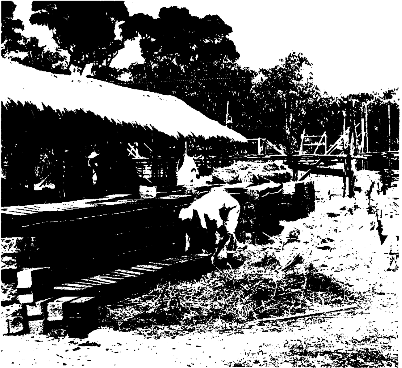
Figure X. 700 Soil-Cement Blocks per Day Were Made in a Hand Operated Machine at Ho Hsiang, Taiwan.
