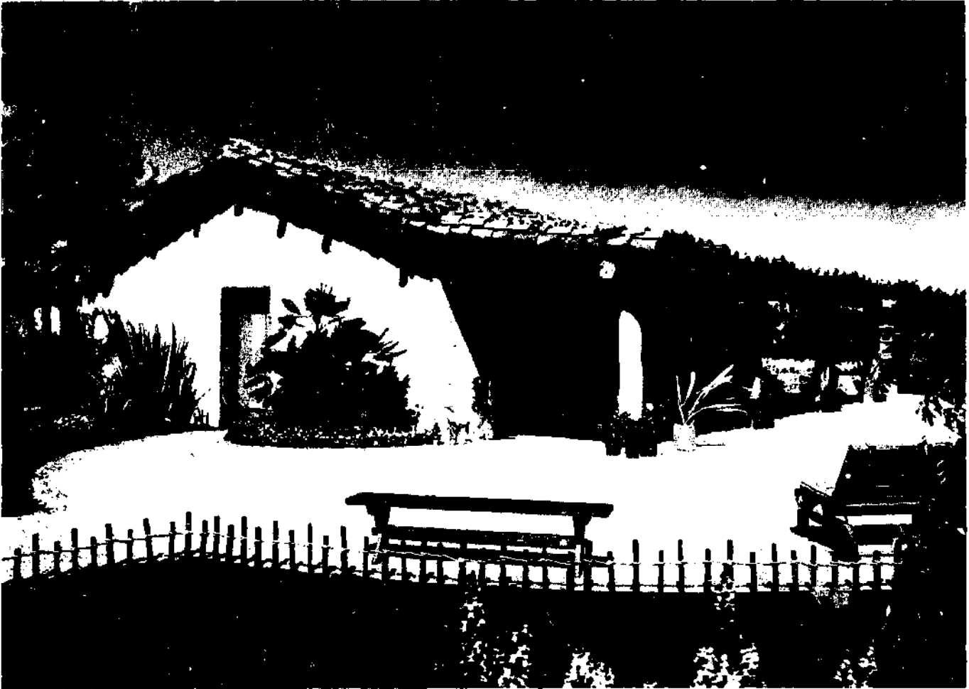
Figure III. A Residence of Stabilized Adobe Brick in North America.
