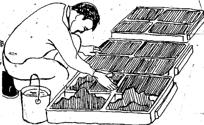
Figure 40. Kneading and leveling the blocks.
