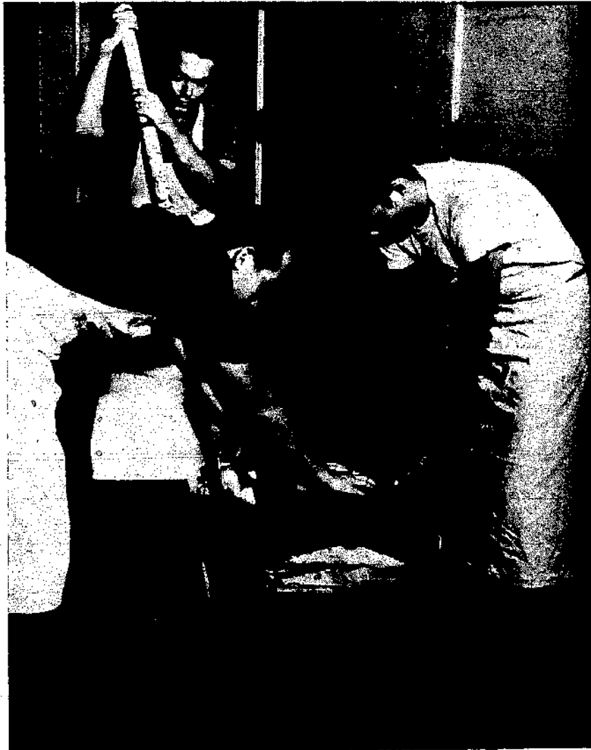
Figure 54. Charging mold box with soil mix.
