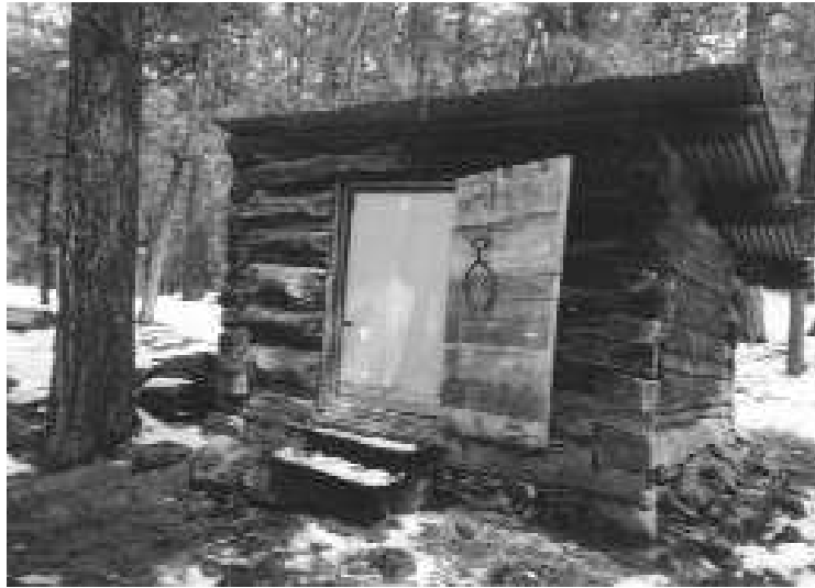
The author's icehouse showing the outside and the inside doors as well as the S-hook holding ice tongs on the outside door
