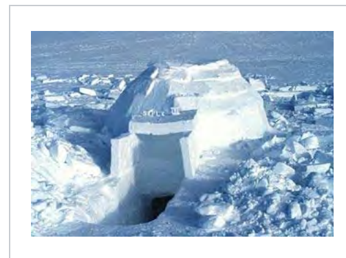
A nearly complete, medium-sized igloo, with excavation under the door and the exterior unfinished
