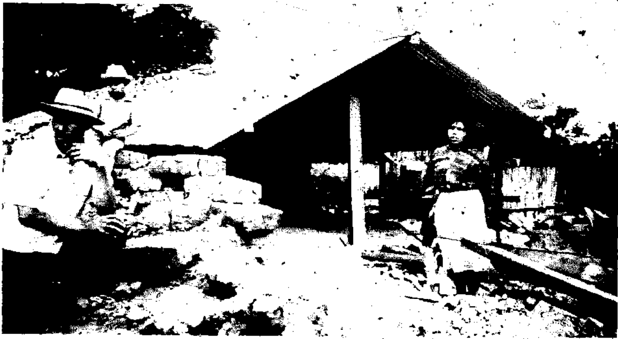
43 A new lightweight roof to replace the heavy tile roof which collapsed during the earthquake in Guatemala
