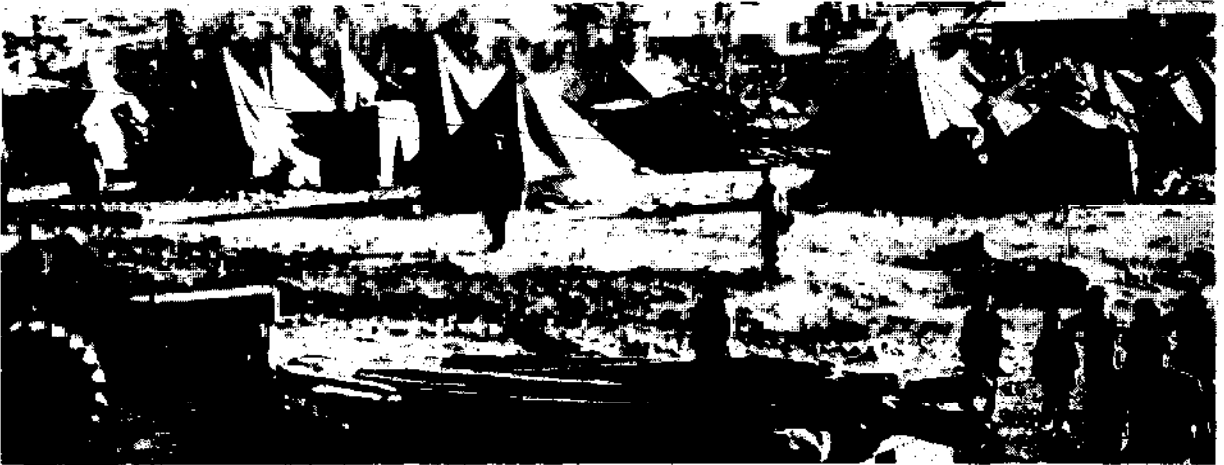
63 Tents provided by Red Crescent in use in Lice, Turkey, eight weeks after the earthquake
