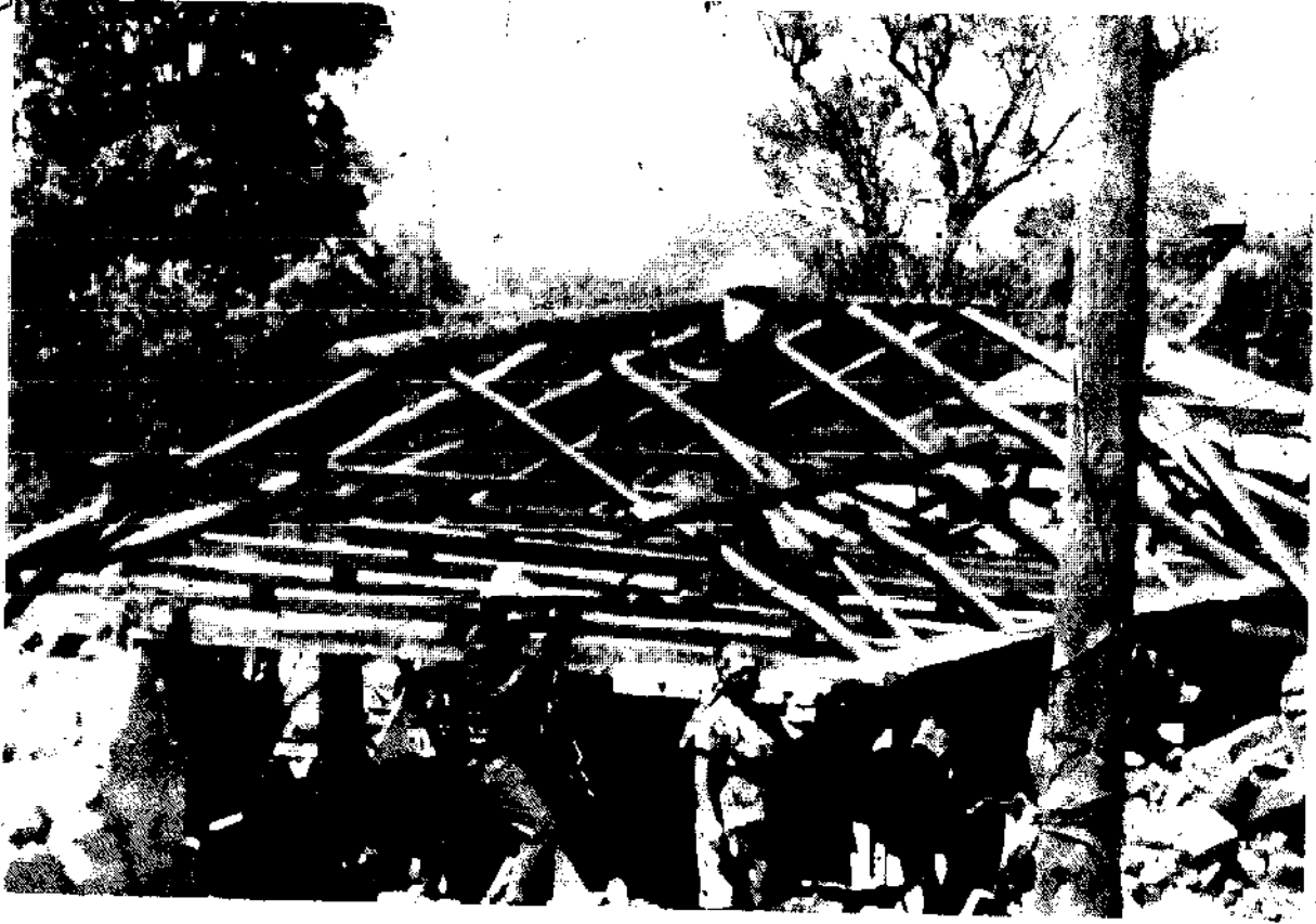
74 Patzicá, Guatemala. A family working on the reconstruction of their house
