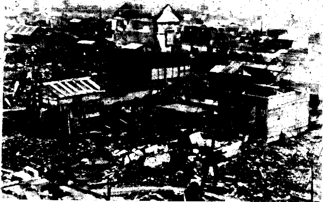
93 Wooden shacks built within scarred ruins following the fire and earthquake
