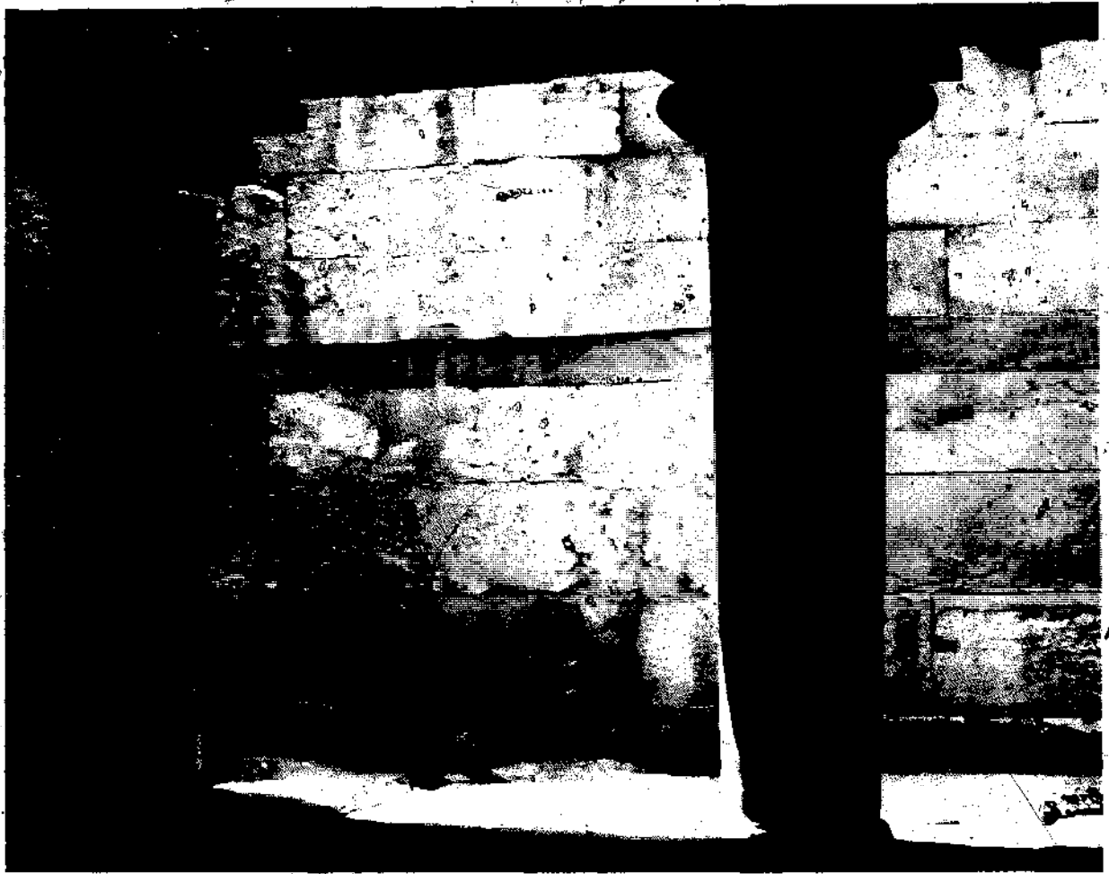
• 11 The Palace of Minos, Knossos, Crete. Note the wooden ring beam on the wall behind the columns
