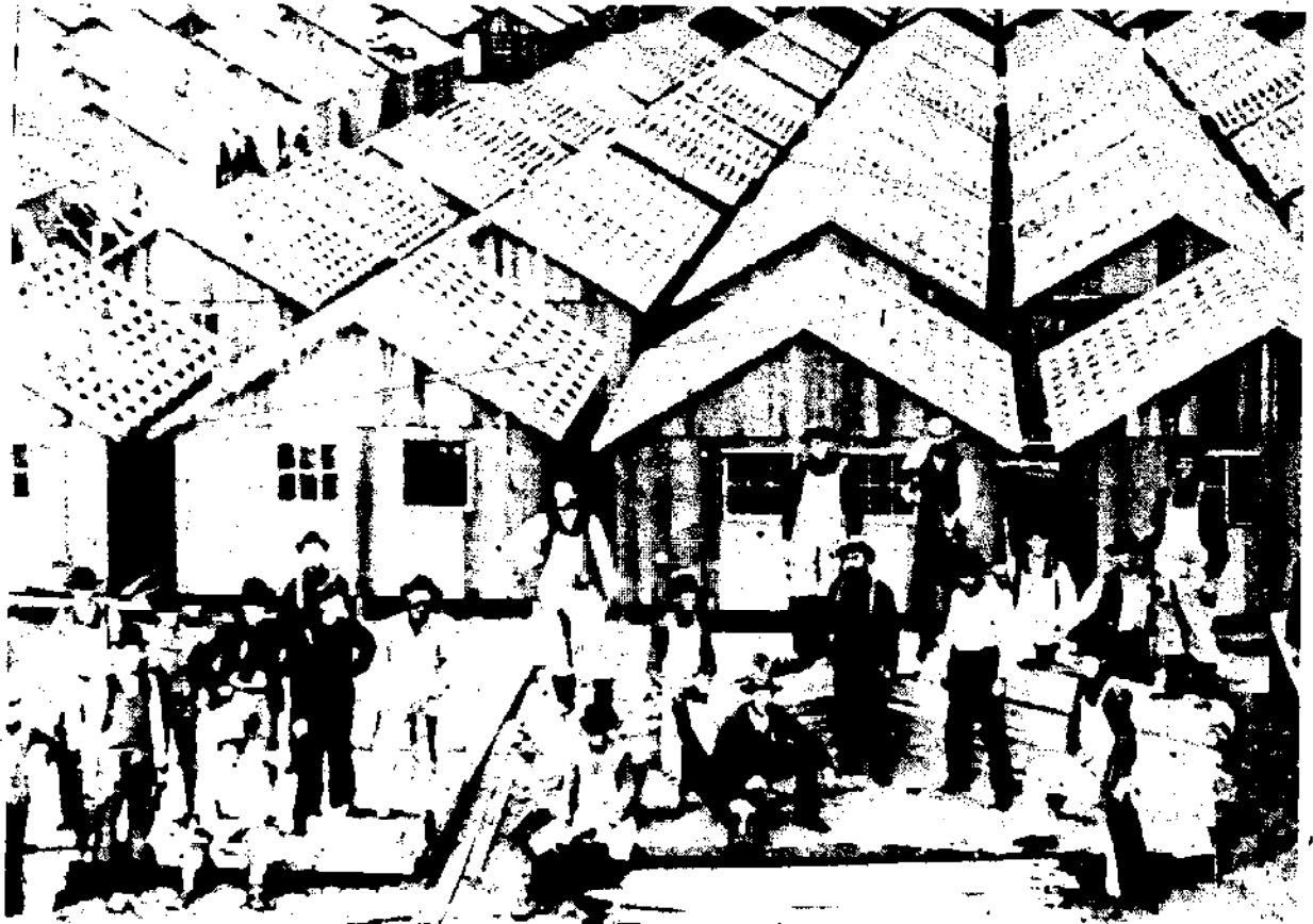
88 5,600 huts were built on this emergency site in Park Presidio Drive.
