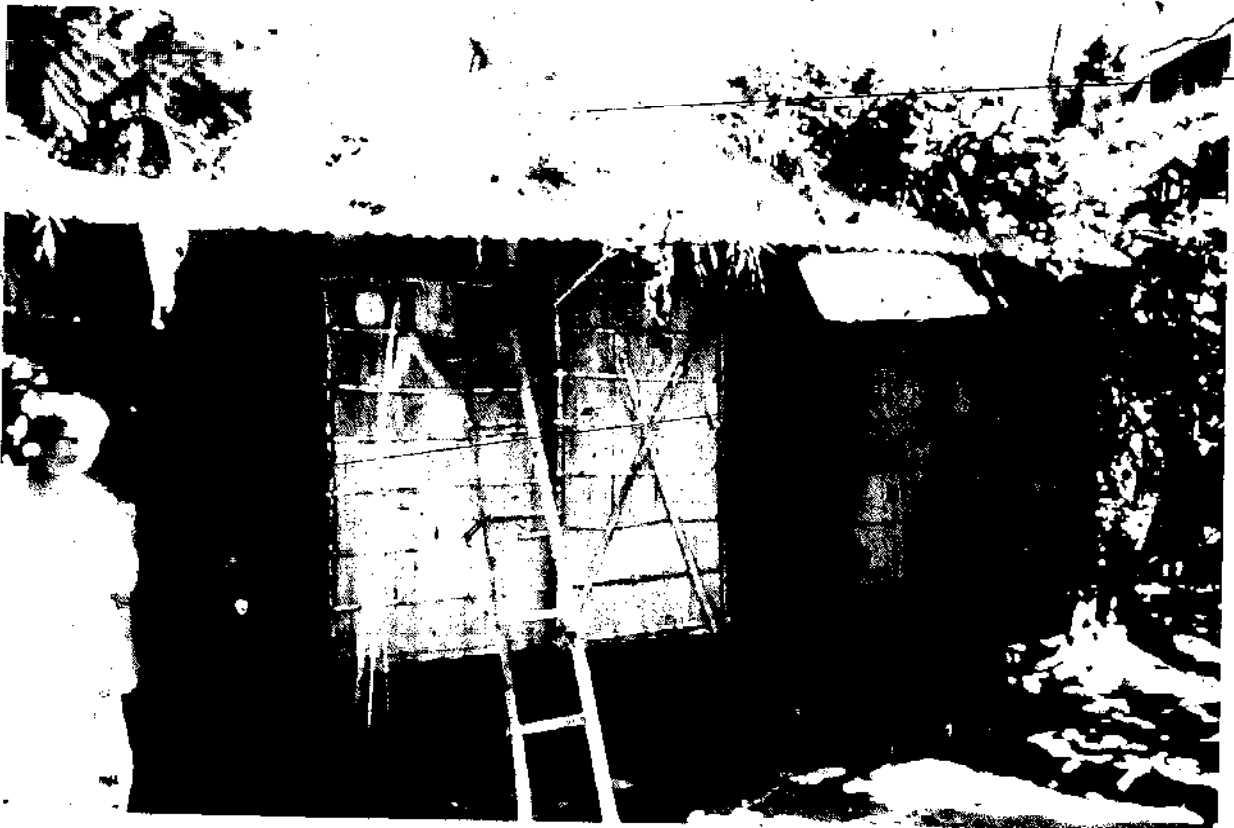
27 House built by EFICOR, a Christian relief consortium in Bangladesh, for a total cost of £52 in 1973. This technique is a development of existing housing techniques in Bangladesh
