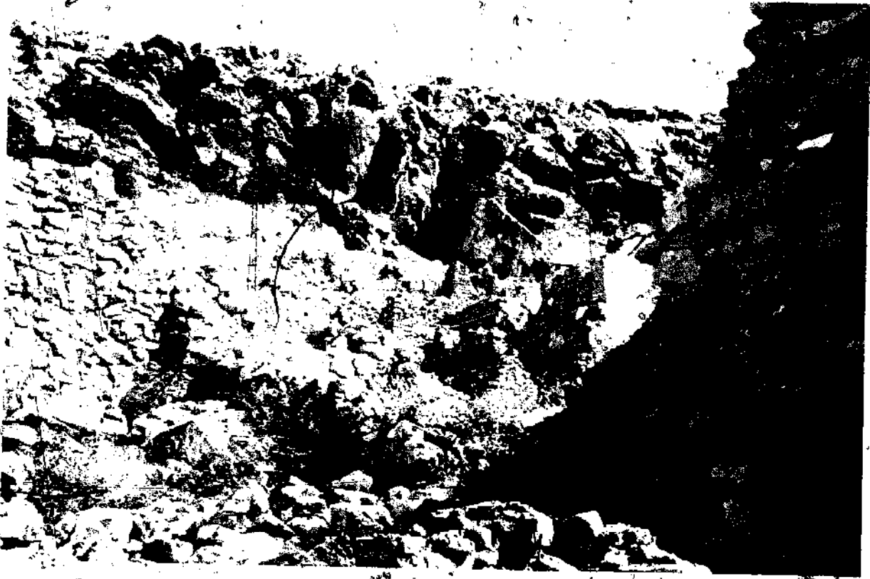
5 Lice, Turkey, following the earthquake of September 1975. Note the vulnerable site below rock formations
