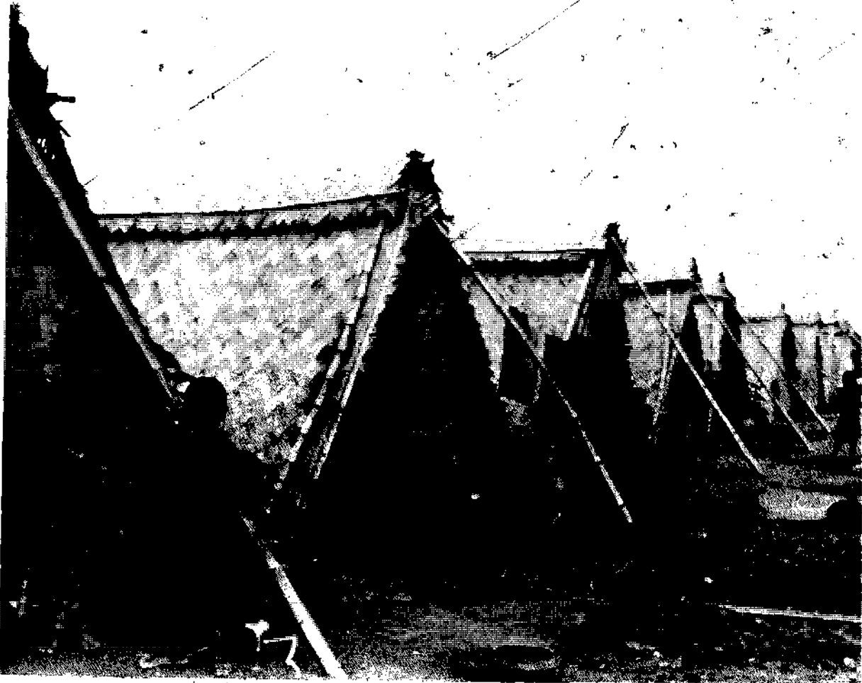
61 Completed 'A' Frame housing at Demra, Bangladesh
