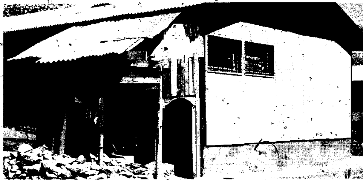
25 Prefabricated housing in Lice, Turkey, as modified by the occupants to give a protected front door and covering for animals
