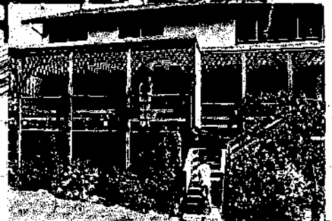
Lowered roof and latticed arches shade west-facing deck from direct sunlight, improve house appearance.
