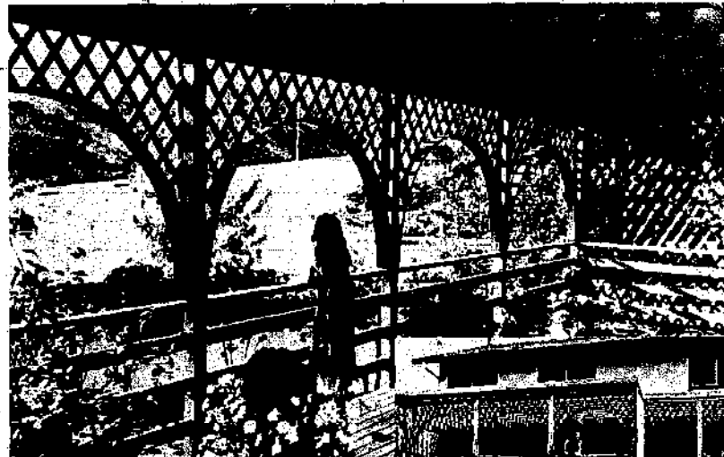
Lowered roof and latticed arches shade west-facing deck from direct sunlight, improve house appearance.
