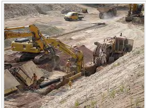
Earthwork in Germany
