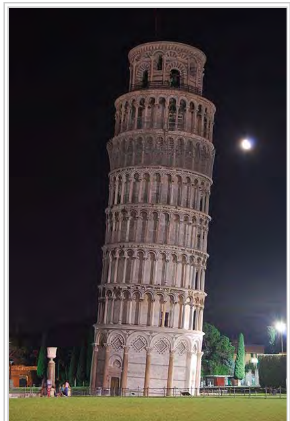
The Tower of Pisa – an example of a problem due to deformation of soil.
