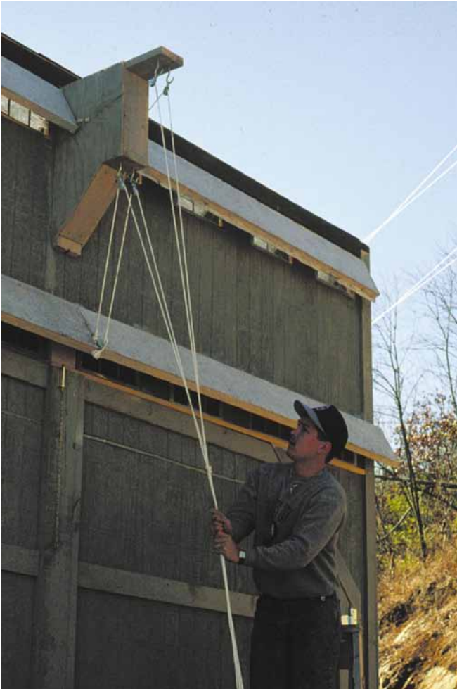
Above: Setting up vent control lines.
