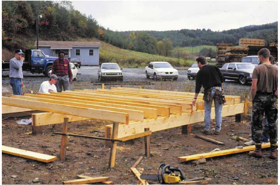
Above: Laying out foundation and floor.
