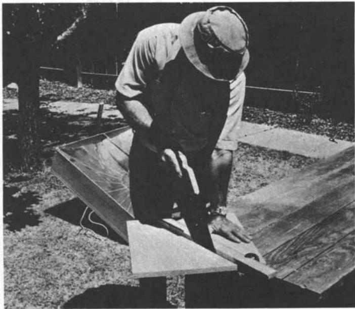
Dan using the clamped board guide to help saw the sides accurately.
