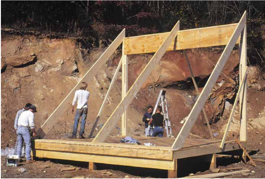
Above: Setting up 2 by 12 south wall rafters.
