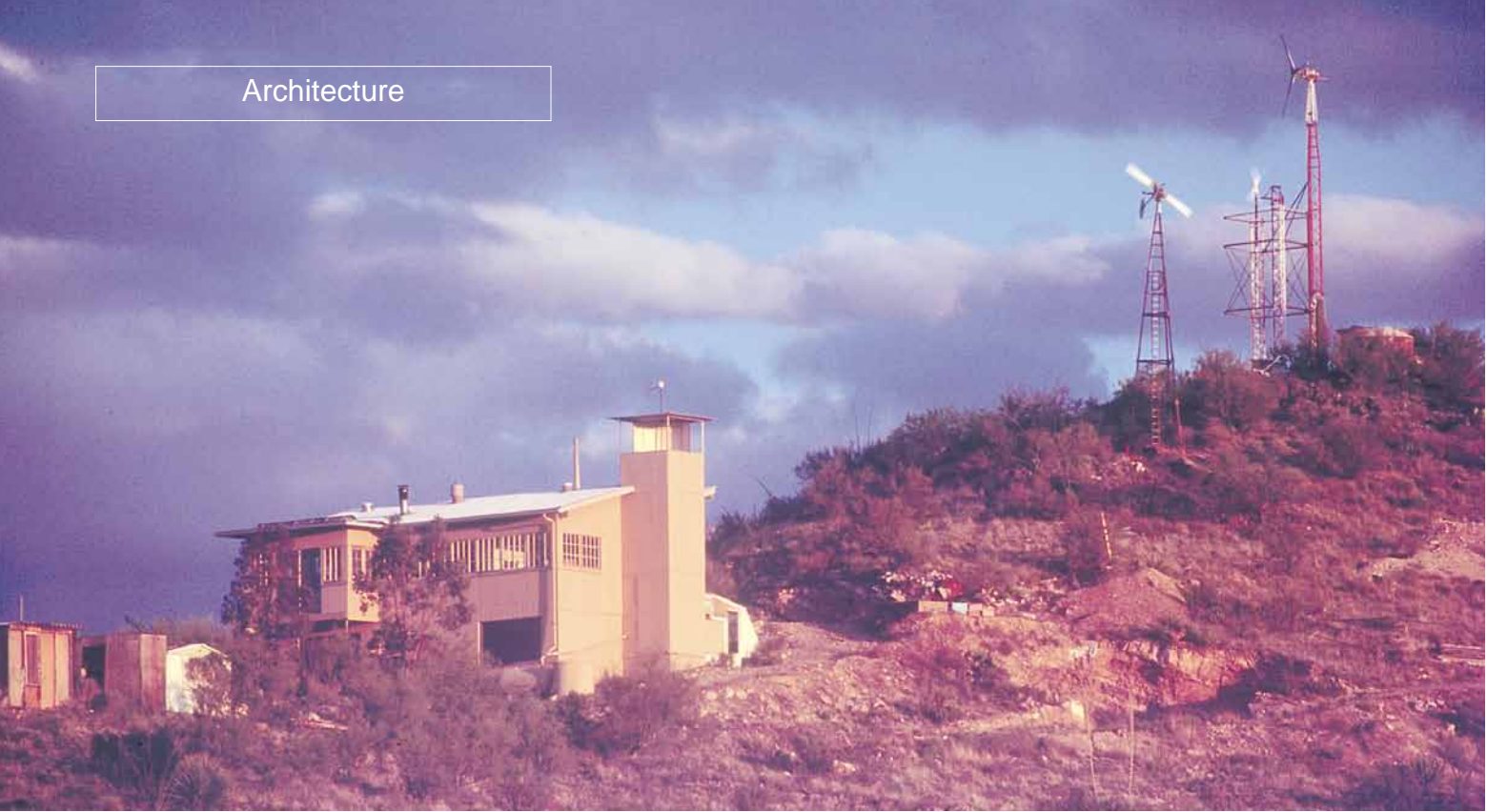
Above: The cool tower keeps Charles Van Meter's house cool all summer long.
