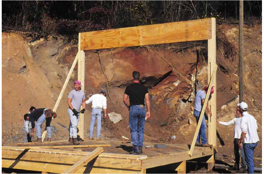
Above: Bracing the north wall.
