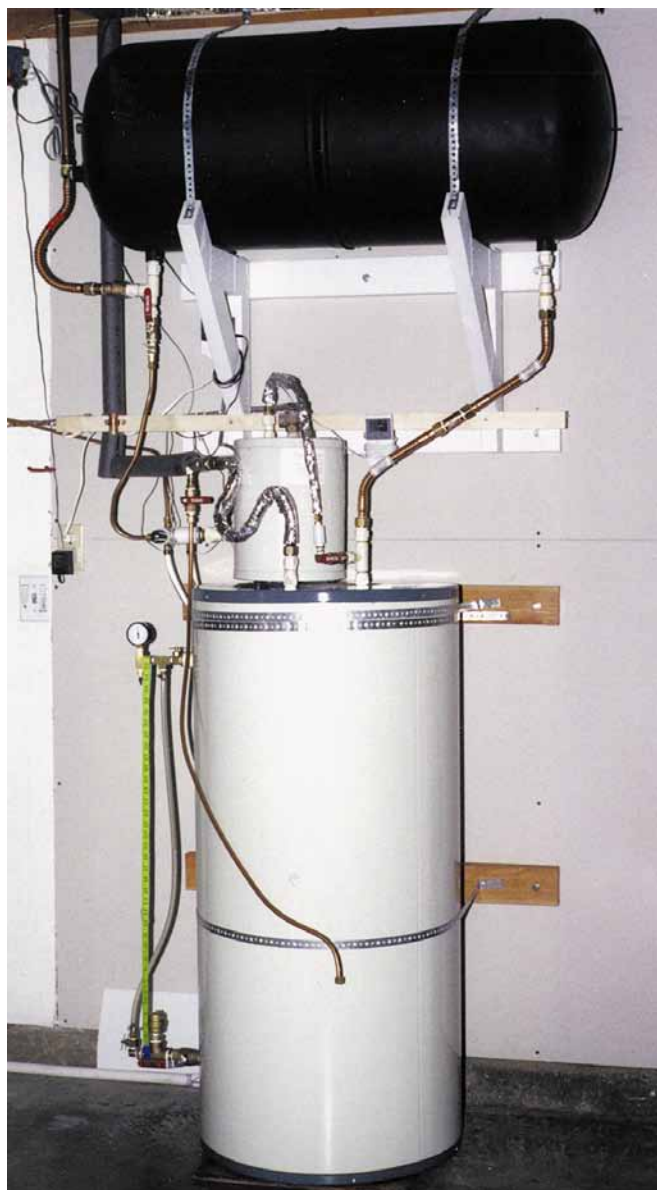
Figure 2: The gravity siphon system.
