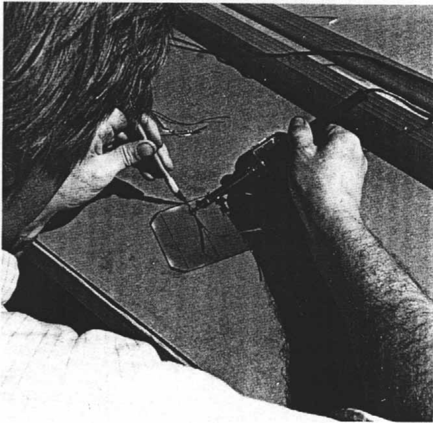
FIGURE 4.4—Soldering copper strips to a solar cell (David Ross Stevens photo).
