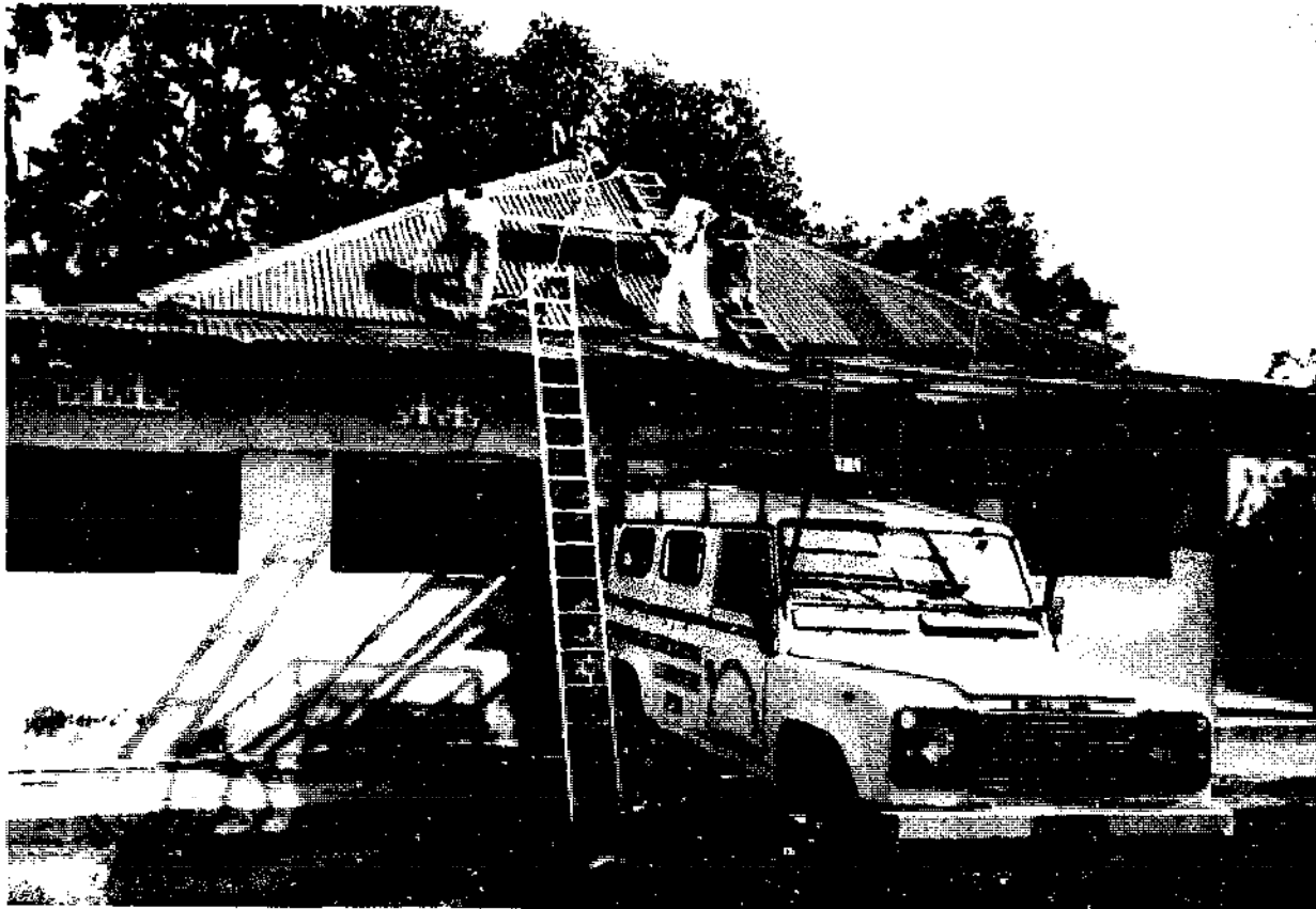
Installing the Solar Array of a Solar Powered Refrigeration and Lighting System for a Health Centre In Zaïre ( I T Power)
