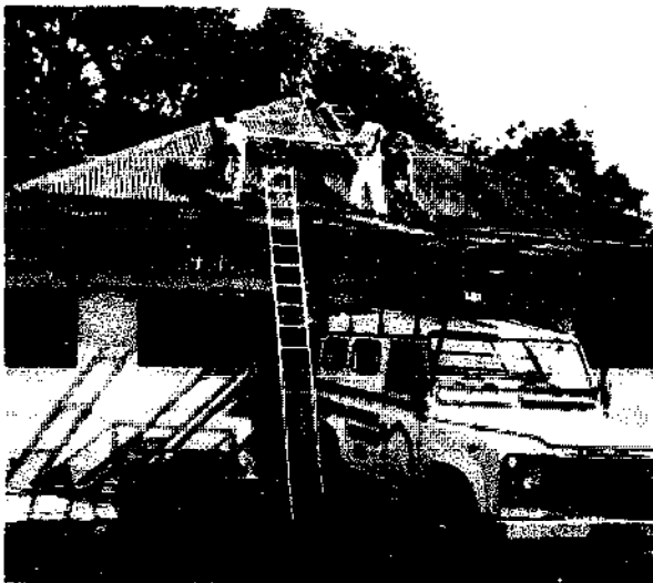
Figure 3.9 Carrying a PV Array onto a Roof
