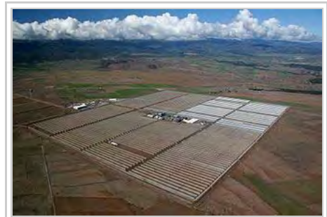
Thermal energy storage. The Andasol CSP plant uses tanks of molten salt to store solar energy.
