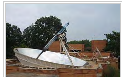
Parabolic dish produces steam for cooking, in Auroville, India
