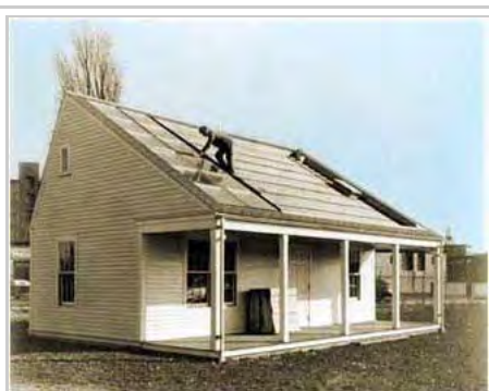
MIT's Solar House #1, built in 1939 in the U.S., used seasonal thermal energy storage for year-round heating.
