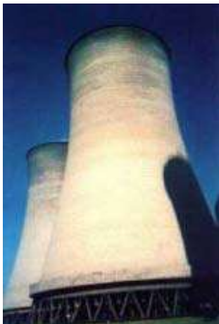
Zambia Cooling Towers Industrial Water Cooling Ltd
