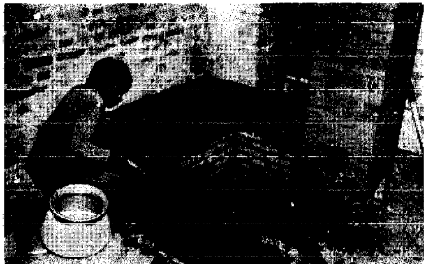
The interior of the stove is lined with a mud-sand mixture.
