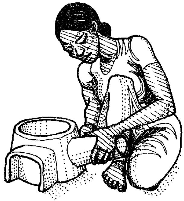
The tunnel is joined to the firebox
