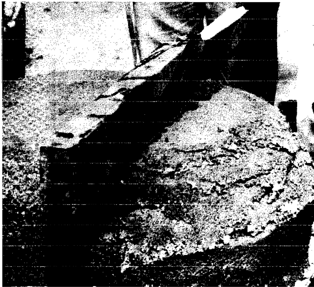
Wet board used to flatten the top of the stove
