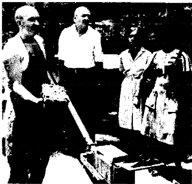
The author and Mr Haas demonstrating the use of a hand press for making briquettes.
