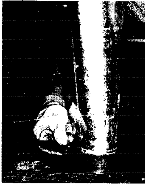
Figure 21.8 —Making the guide mark on the crimped end of the adapter. The pipe will be allowed to expand slightly to ensure a tight fit.
