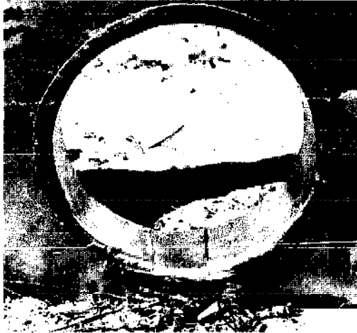
Figure 13.16—Stokehole collar after mounting, inside view. (The gap at the bottom was caused by an error.)
