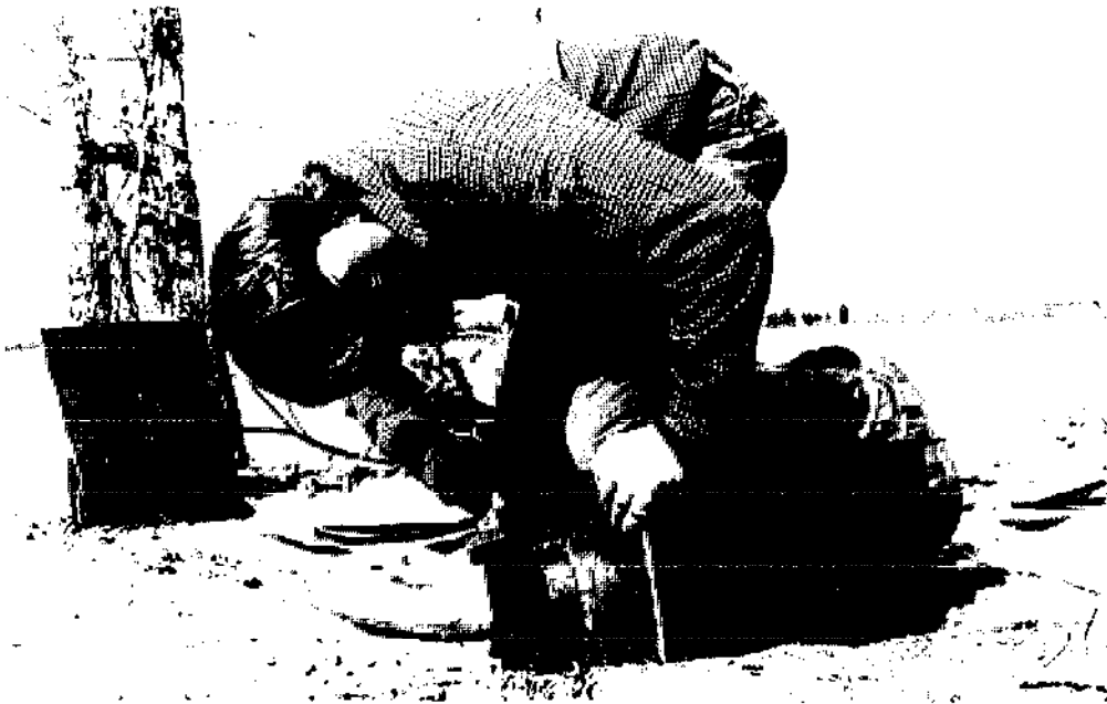
Figure 13.17—Mounting the stove bottom.
