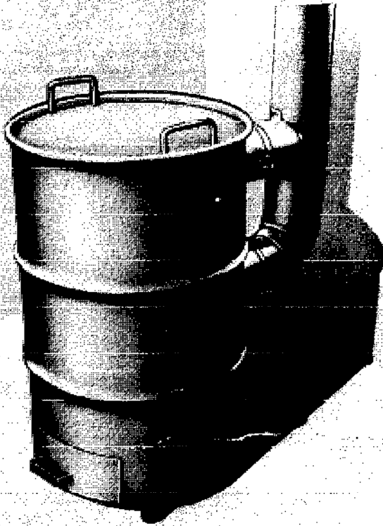
Figure 1.—The double-drum sawdust stove.
