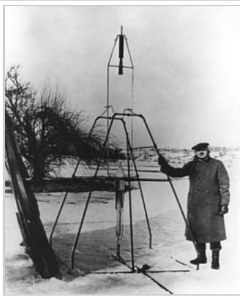
Goddard with a liquid oxygen-gasoline rocket (1926)
