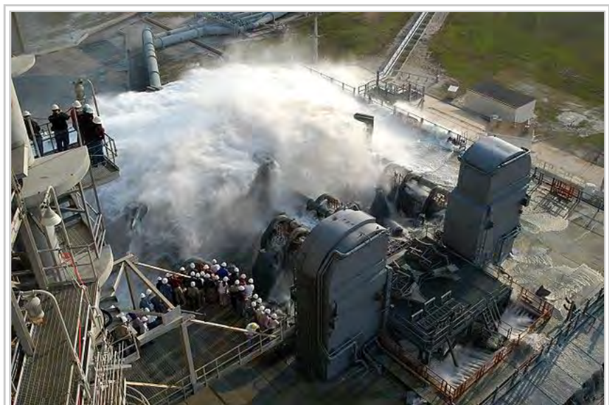
Workers and media witness the Water Sound Suppression System test at Launch Pad 39A.
