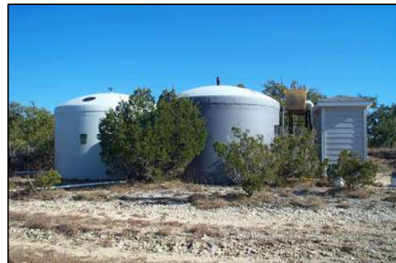
Figure 2-5. Two 10,000-gallon fiberglass tanks
