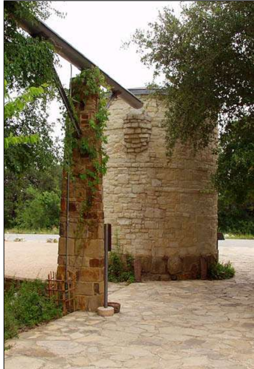
The entry cistern at the Lady Bird Johnson Wildflower Research Center is reminiscent of the stone-and-mortar cisterns used by Hill Country settlers. Water from a 1,200-square-foot roof area is conveyed to the entry cistern via an aqueduct.
