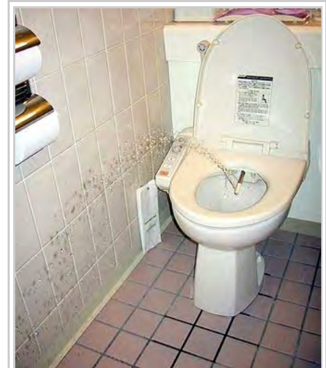
A Japanese bidet spraying water from its jet. The water jet is used to wash the anus and buttocks after defecation.
