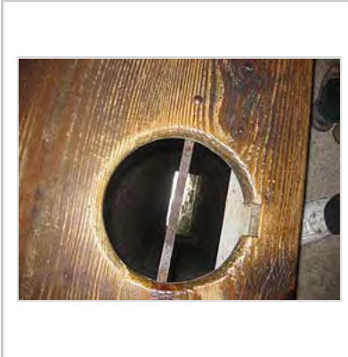
View looking down into garderobe seat opening
