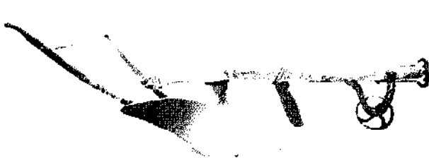
From the 1830s to the 1860s, the Eagle plow was the most popular tillage implement in the United States. This plow was built in many styles, but it was characterized by a longer and more curved moldboard than that found on other plows. The Eagle plow was well suited for turning a furrow in most soils. (Smithsonian Institution.)
