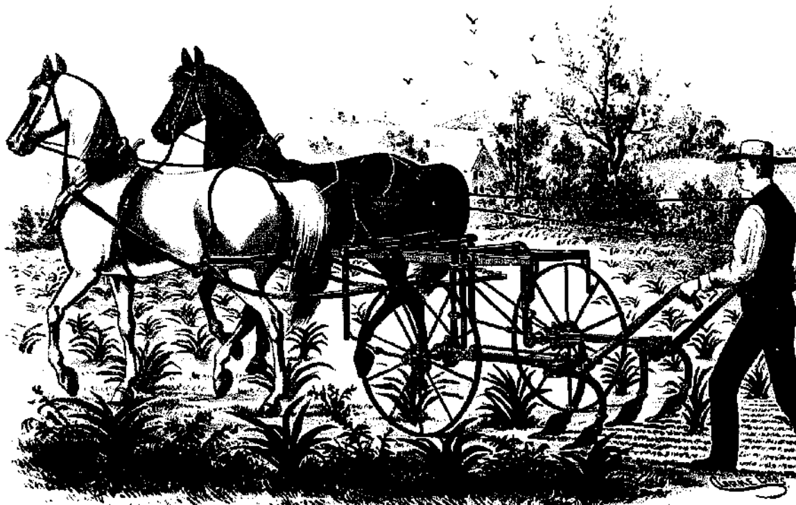
The P. P. & Mast Company of Springfield, Ohio, manufactured the No. 4 Buckeye Sunbeam Walking Cultivator. This implement was designed with a high frame and an arched axle to pass over waist-high corn plants.
