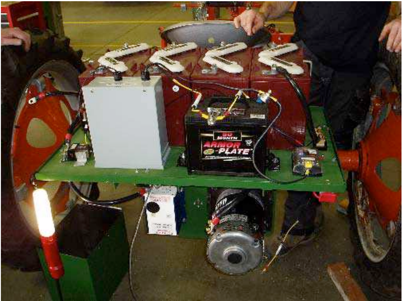
Battery rack and battery bank installation.
