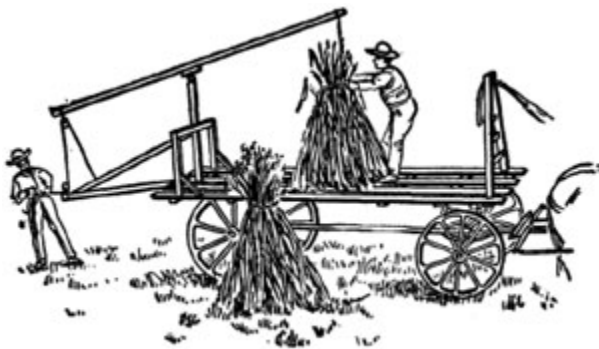
LOADING RIG IN USE
