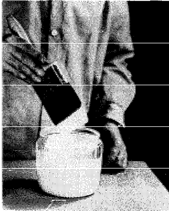
Fig. 11.5. In painting, dip the brush in the paint about one-third the length of the bristles.
