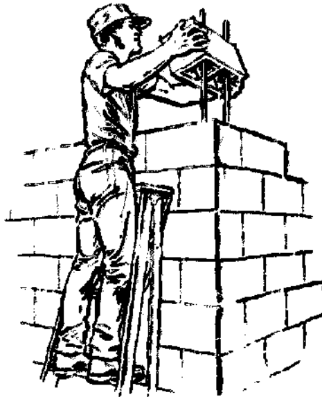
Fig. 32.7. Stacking a concrete block wall without mortar for surface bonding.
