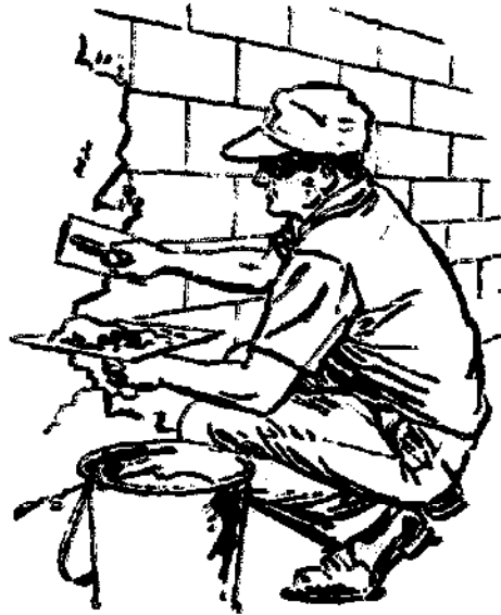
Fig. 32.6. Surface bonding of a stacked, mortarless, concrete block wall.
