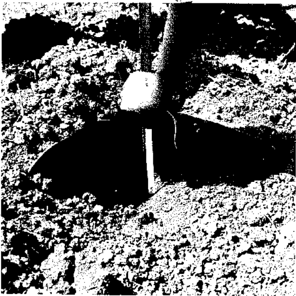
After moving about 5 m check the depth of working.
