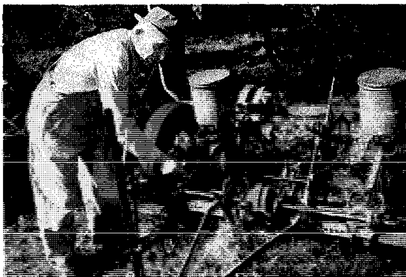
Louis Suchy with his check-row planter. Here he points to the trip mechanism which is engaged when buttons on the guide wire pass through the checkhead. Ron Krupicka
