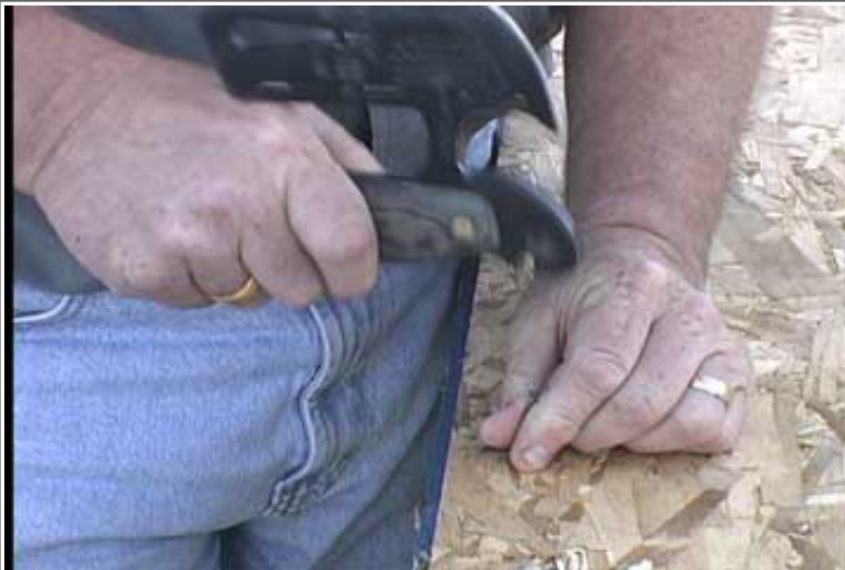
The back of the tool finds use as a hammer and pounds in a nail.
