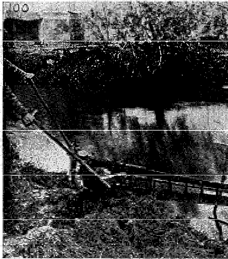
FIG. 79. CHINESE MAN-POWER IRRIGATION APPARATUS WORKED BY THE HANDS.
