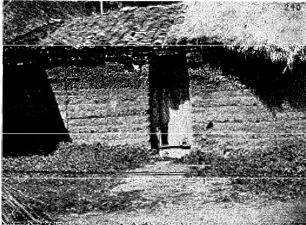
FIG. 436. A CHINESE HOUSE BUILT OF PISE DE TERRE.
