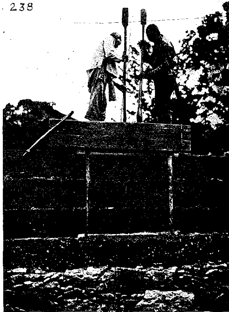
FIG. 440. BUILDING A WALL OF PISÉ DE TERRE AT KULING, SHOWING THE POSITION AND END LOCKING OF THE FORM AND ONE OF THE WALLED-IN WINDOW FRAMES.
