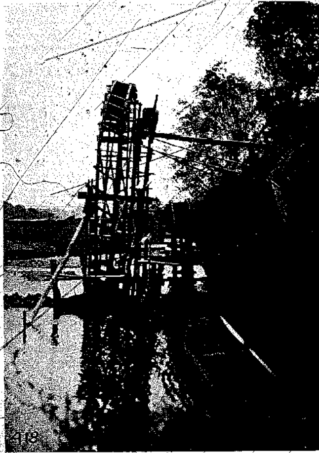
FIG. 175. UNDERSHOT WATER-WHEEL FOR RAISING WATER.
