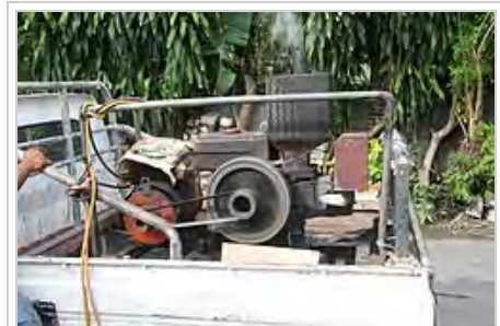
A diesel powered welding generator (the electric generator is on the left) as used in Indonesia.
