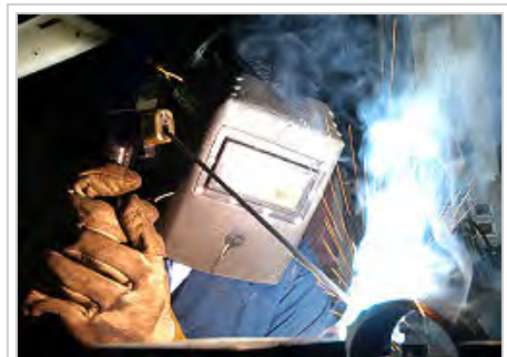
Shielded metal arc welding
