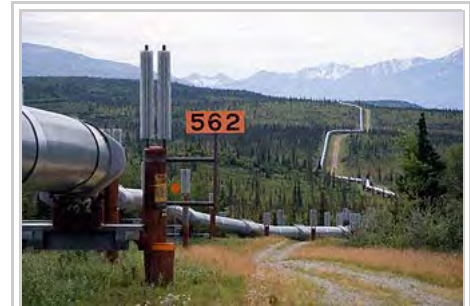
Trans-Alaska Pipeline for crude oil
