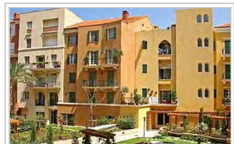
The main square of Saifi Village in Centre Ville, Beirut, Lebanon
