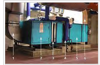
Air handling unit, used for heating, cooling, and filtering the air
