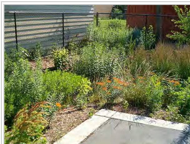
Business parking lot that drains to a rain garden. The curb retains the asphalt pavement, yet lets water flow off the edges.
