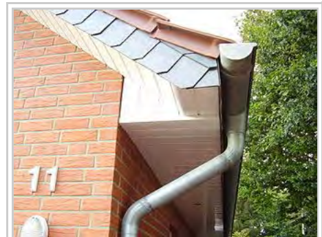
Eaves gutter and downpipe
