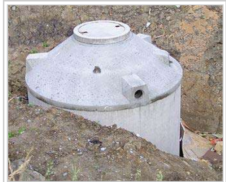
A cistern for rainwater storage
