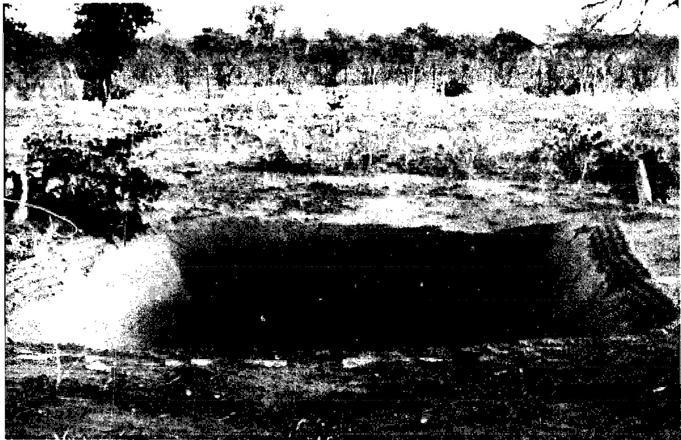
Plate 5. An excavated rainwater tank at Tamasane, Botswana, built in 1968, replastered in early 1970s and still operating in 1983. It is used to irrigate a school garden (see pages 92-3). The absence of a fence or cover can be dangerous — even tragic.
