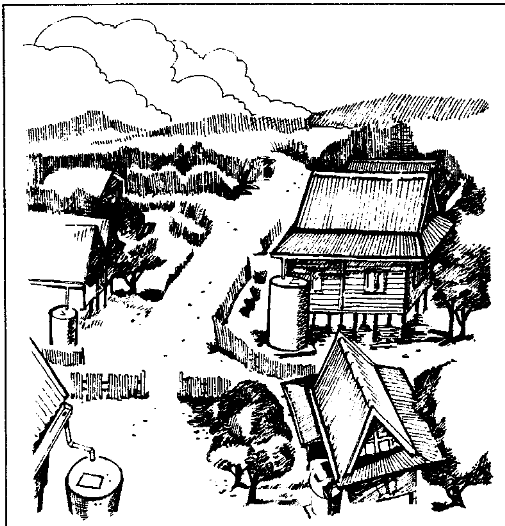
Fig. 4.1 Raised wooden platform houses with corrugated iron roofs in Khon Kaen Province, Thailand. Gutters are usually attached to only one slope of the roofs. The houses have bamboo-reinforced concrete rainwater tanks such as those built within the programme described in the text. See also Table 4.1. This illustration is from a booklet distributed in Thailand by UNICEF. (UNICEF and Fricke 1982)
