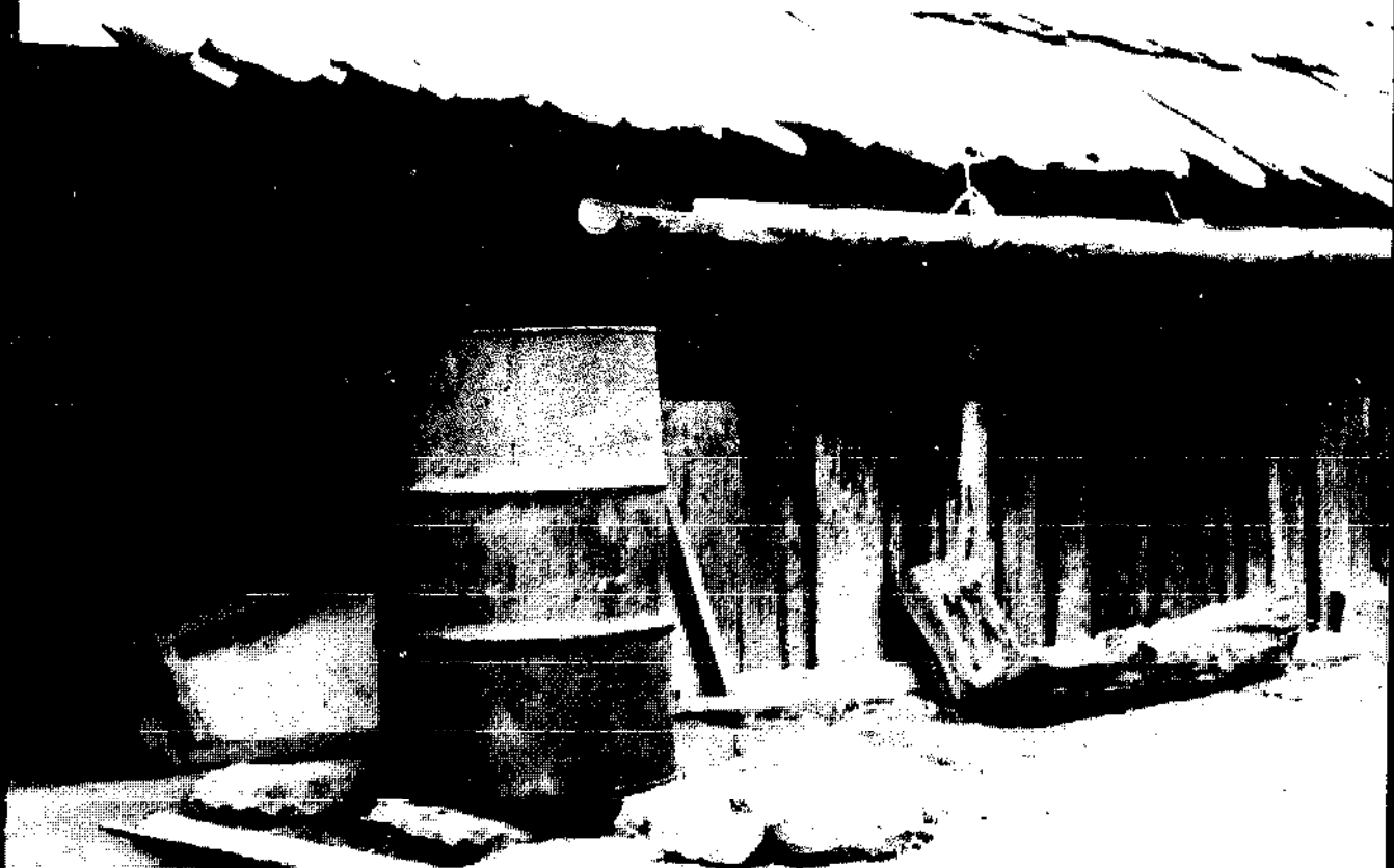
Plate 2. A very basic domestic system in Thailand — a split (halved) bamboo gutter directing runoff from the roof (wooden tiles) into an old oil drum. (John Collett)
