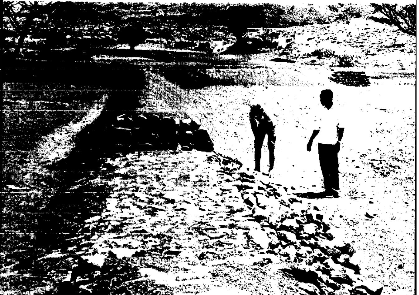
Plate 14. Detail of gabion spillway construction in a bund system — part of the River Naupwala water harvesting scheme, near Lokitaung, Kenya.
