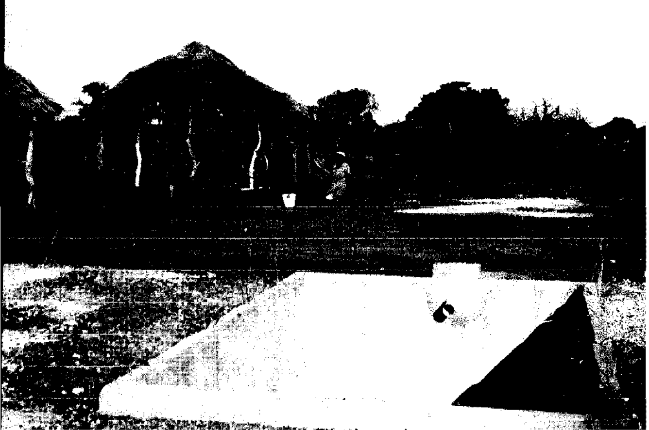
Plate 8. A brick and cement rainwater catchment tank at Pelotshetla. In the background a woman can be seen smearing the threshing floor catchment apron with a mixture of dung, water and mud. (John Gould)
