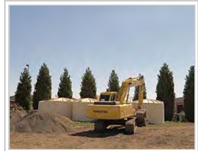
Large polyethylene rainwater tanks being installed.
