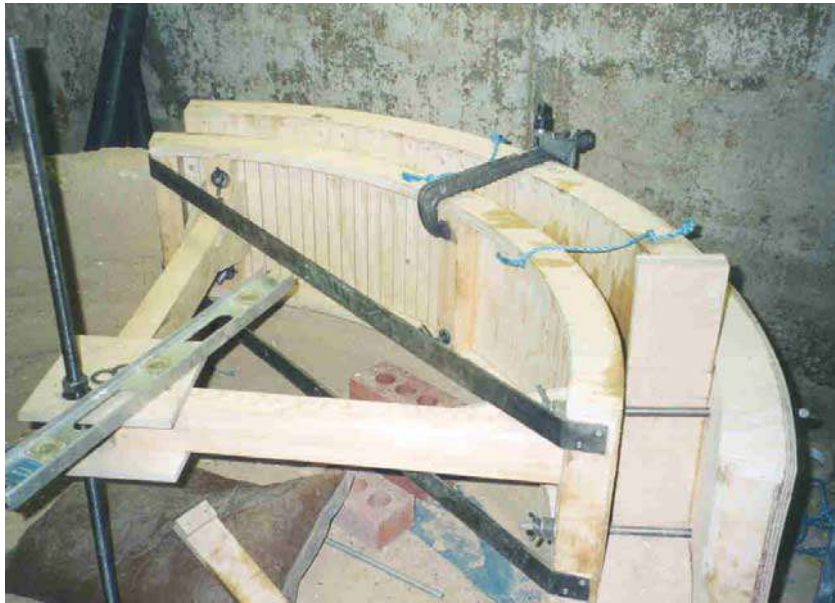
Figure 7.3 – Shuttering manufactured in the UK
