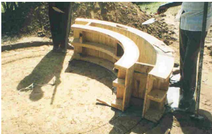
Figure 7.4 Shuttering manufactured in Uganda
