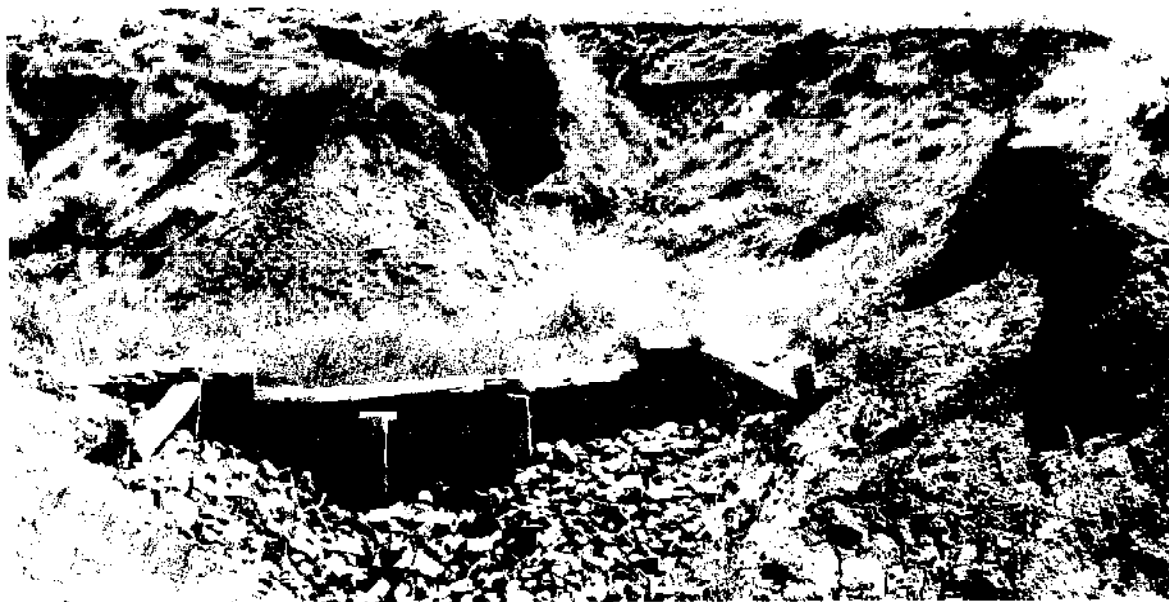
Figure 4. Conservation measures often may rely on local materials and hand labour, for example, in gully correction work with small logs and rocks (Photo courtesy of U.S. Forest Service).
