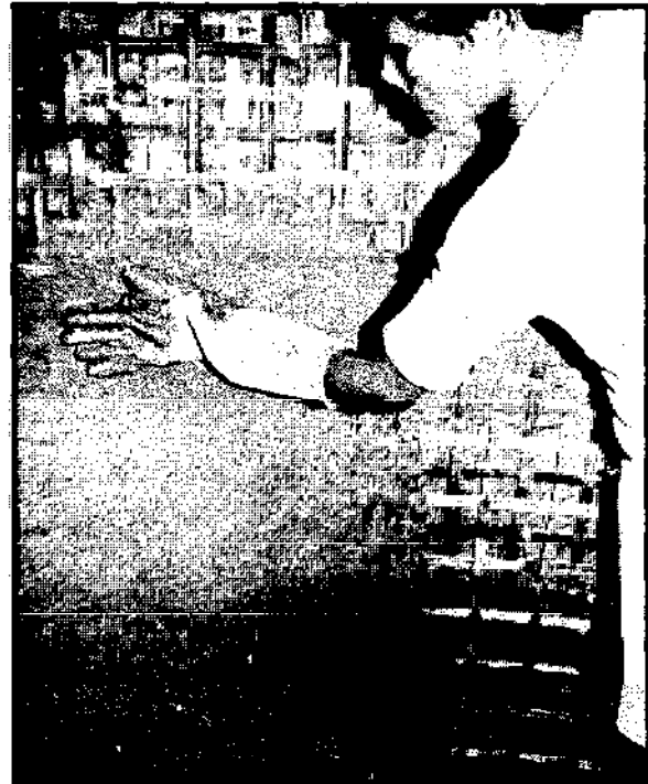
Left: internal plastering of the tank floor Right: applying plaster with rubber gloves
