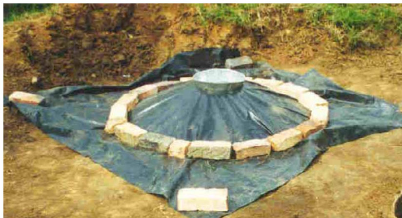
Figure 2 Mould ready for the cement render
