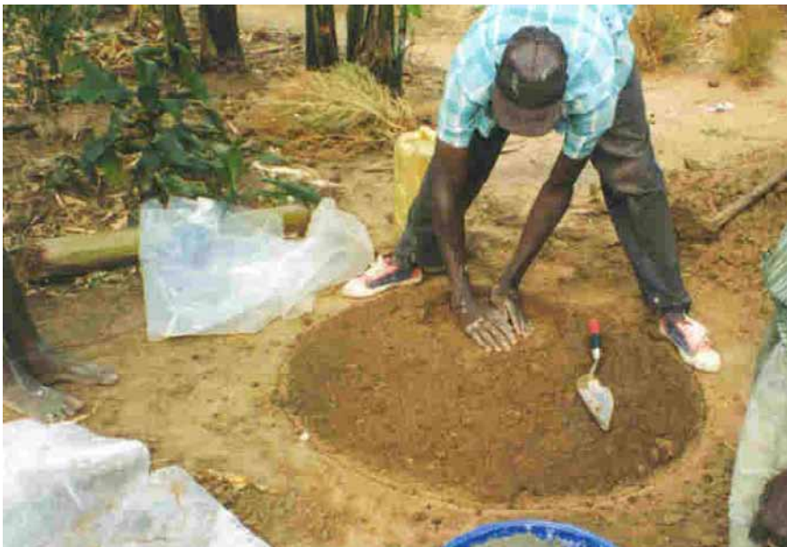
Figure 1 Mould for brick jar cement cover
