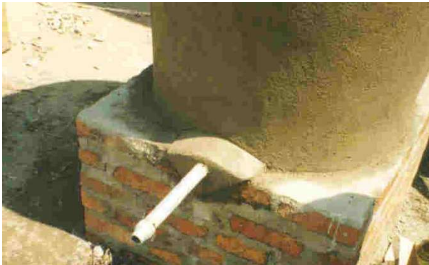
Figure 5 Detail of the outlet fixing
