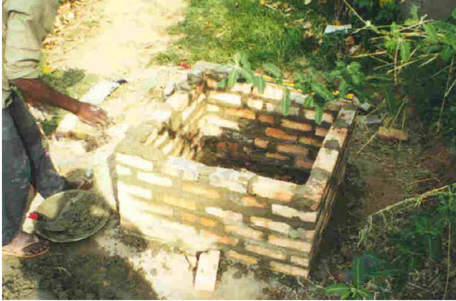
Figure 1 Brickwork plinth
