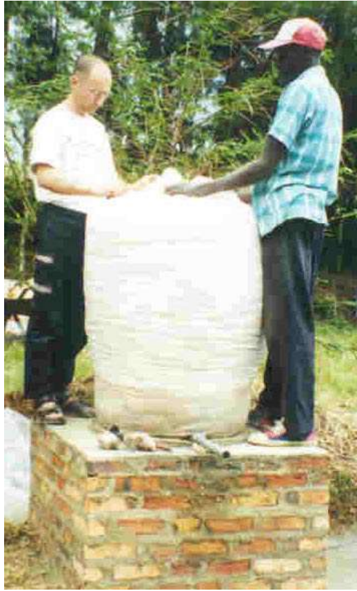
Figure 2 The filled polypropylene sack mould
