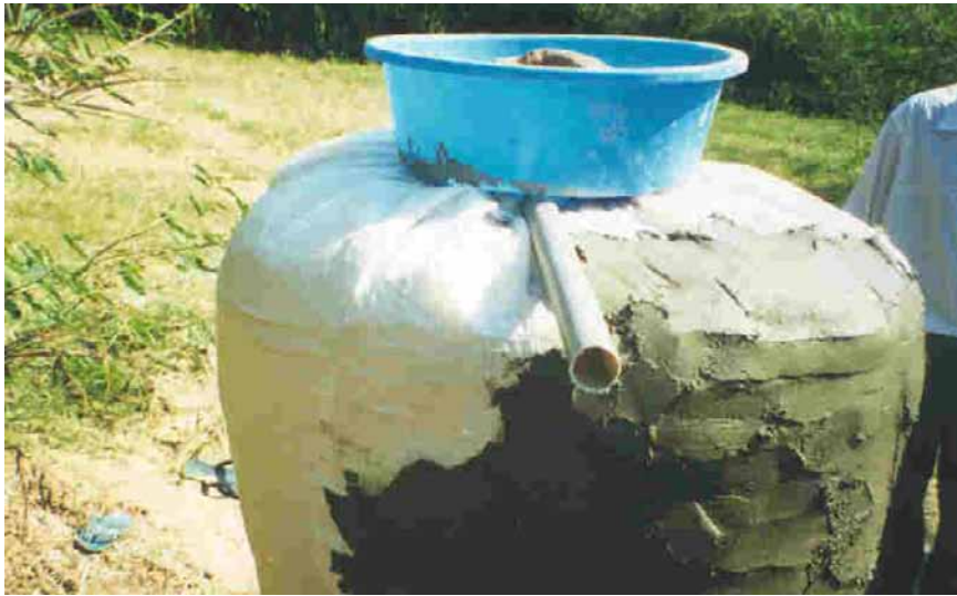
Figure 3 Overflow, filter basin and first coat application
