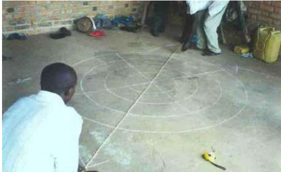
Figure 3 – Marking out the hoop diameters before bending
