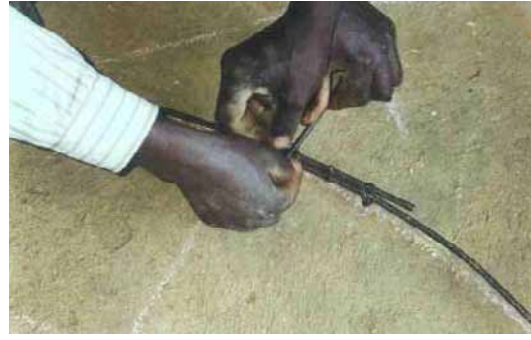
Figure 4 – Tying the hoops using tie wire and a nail
