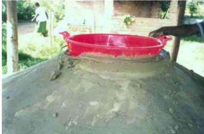
Figure 16 – showing the lip being built up around the basin – note the steel hoop in place
