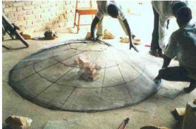
Figure 13. Applying the chicken mesh.
