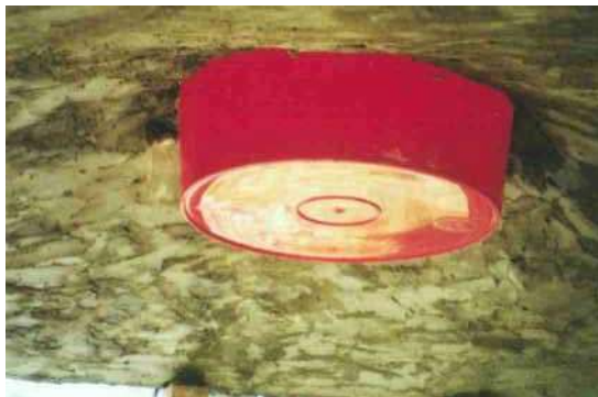
Figure 17 – Showing the underside of the cover after rendering is completed
