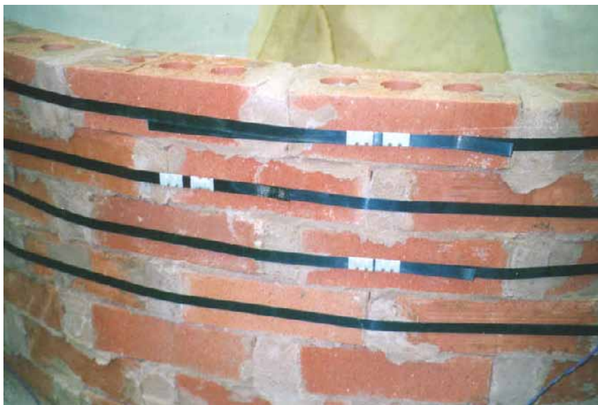
Strap showing crimps
