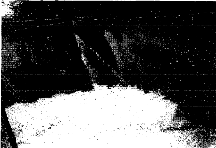
Figure 13.6. Hydraulic jump for rapid mixing (Philippines)
