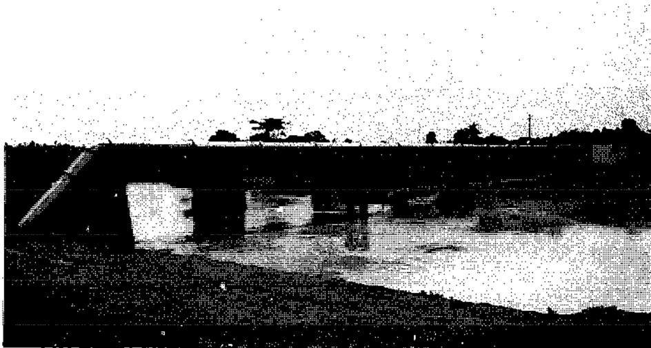
Figure 18.8. Water transmission main river crossing
